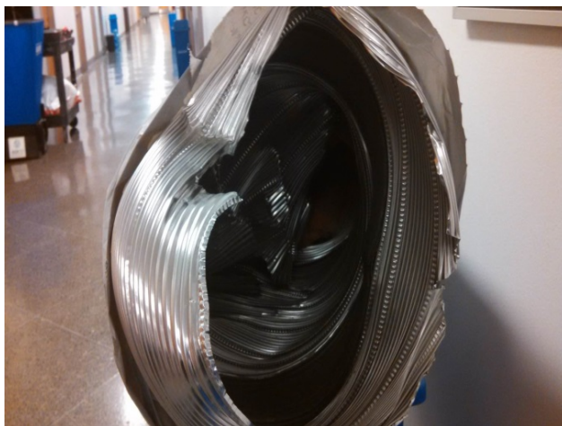
Aging HVAC Systems (Damaged Duct)
